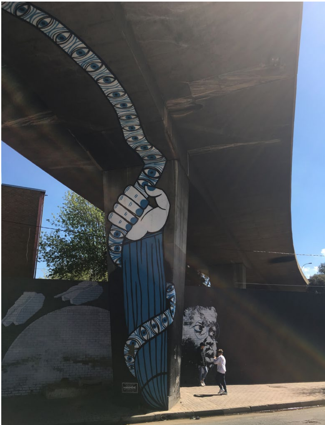
Figure 2: The graffiti work 'snakes' around the structure of the road flyover, Maboneng.
