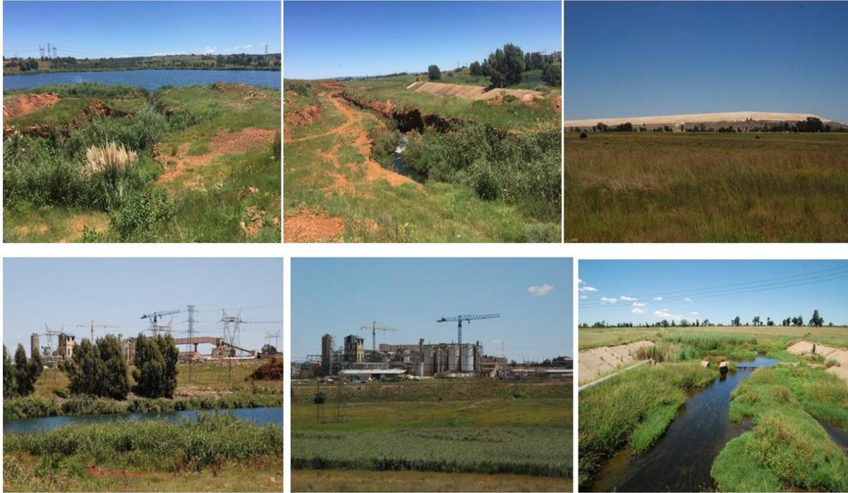
*Figure 69: Wonderfonteinspruit showing flows bypassing the Cooke Attenuation Dam, and the flow diversion offtake structure with limited flood capacity further downstream.*
