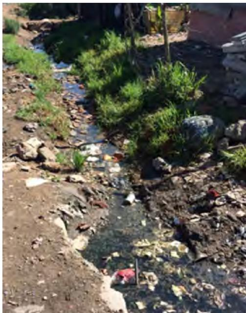
**Figure 4.18:** Large clogged stormwater drain running through the rubbish dump and into the river
