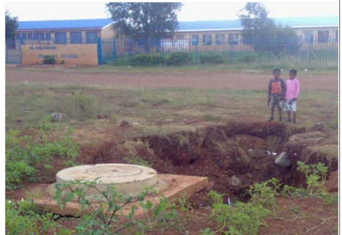
Sink-hole caused by leaking infrastructure in Khutsong near Carletonville (Courtesy: Eric Stoch (Stoch Environmental), 2011)
