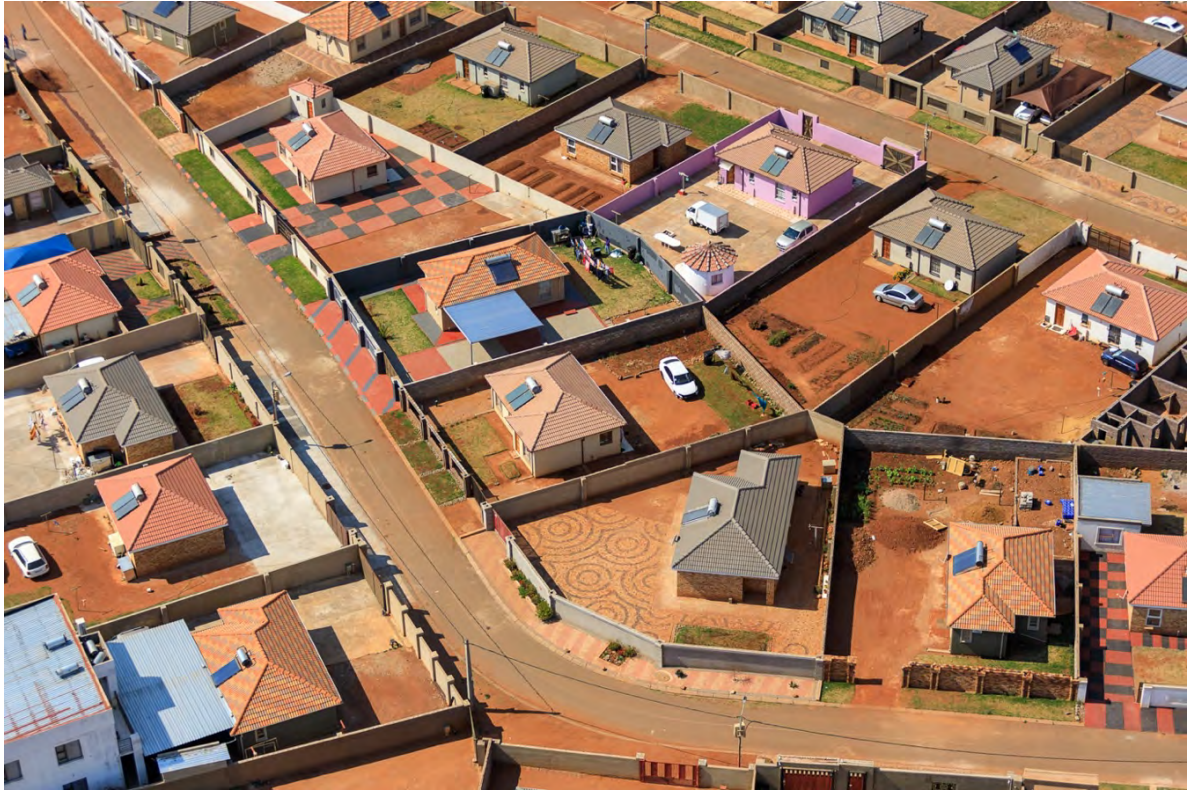
Figure 3.3: Bonded houses on their own stand in Lufhereng Phase 1. Photograph: Clive Hassall, 2021.
